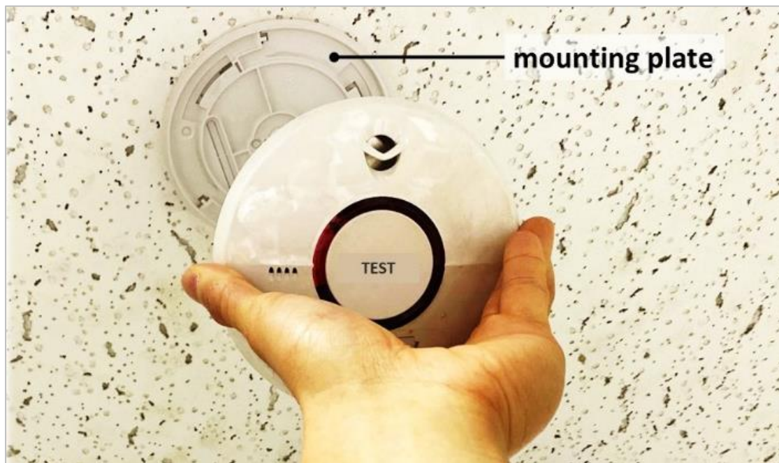
Figure 2 – A stand-alone fire detector being mounted onto mounting plate
